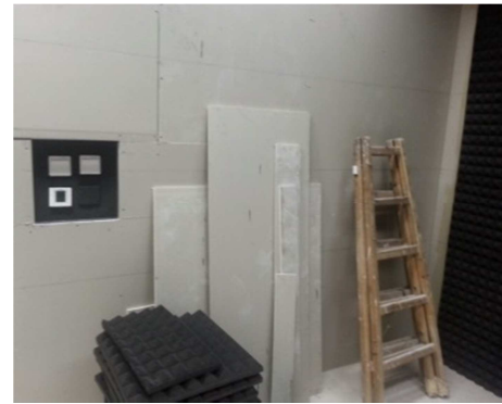
Figure 6. Panel Absorbers was stuck on the surface of plaster board.
