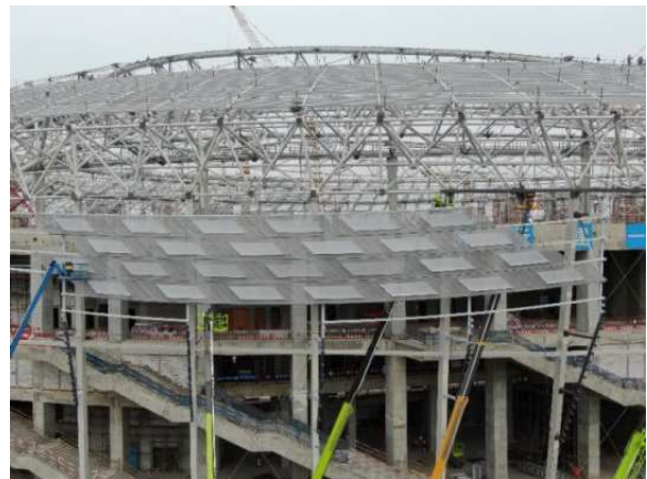
Figure 35. Installation adjustment of real sample panels.
