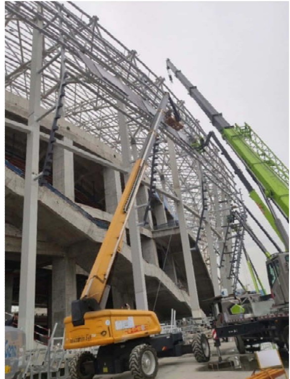
Figure 34. Hoisting of real sample panels for on-site installation.
