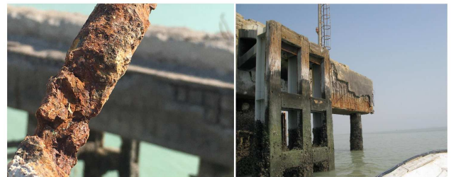
Figure 1. An image of rebar corroded (a) rebar and (b) piers of the P3 & P4 piers of Imam Khomeini petrochemical.
