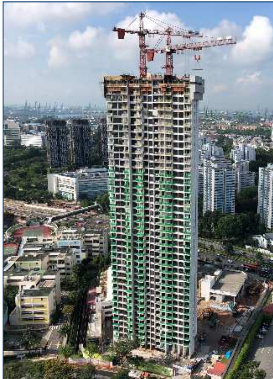
Figure 21. Completion of module installation (April 2018).
