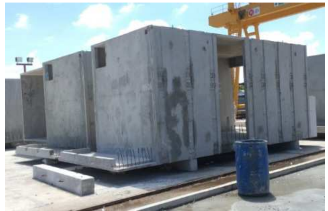
Figure 13. Completed PPVC concrete carcass.
