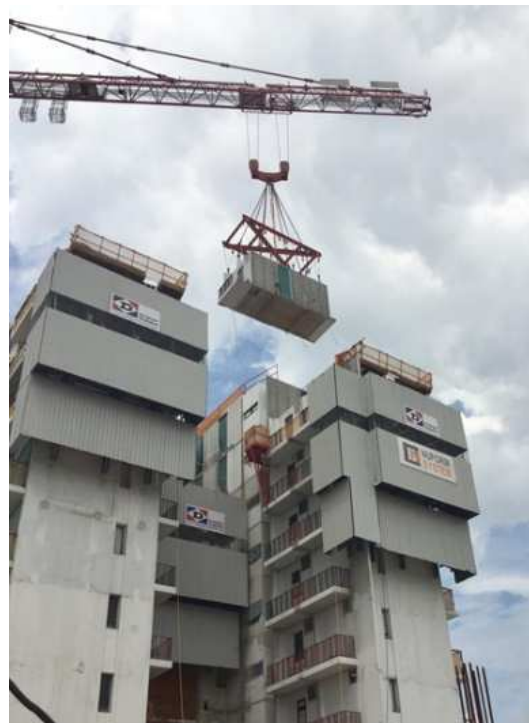
Figure 18. Hosting of module.
