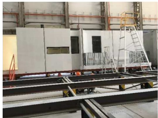
Figure 16. Trial fitting of modules for a residential unit.
